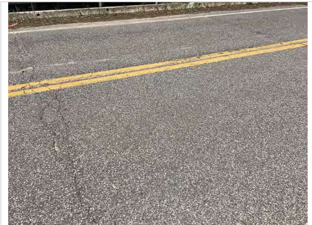
Span 2 view across deck
