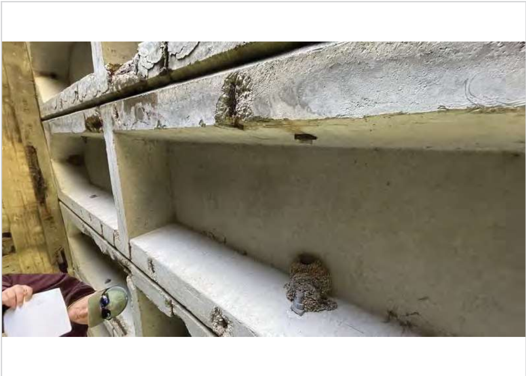
Bottom deck span #2 PCCS "C"
