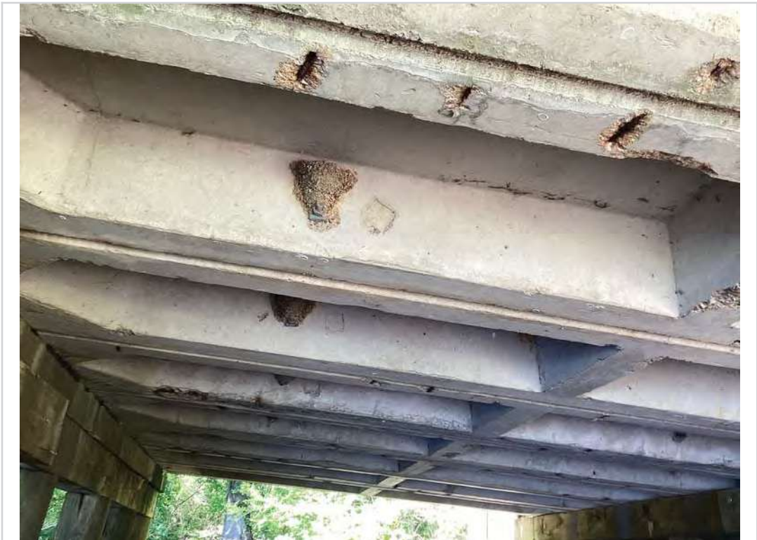
Bottom deck span 3
