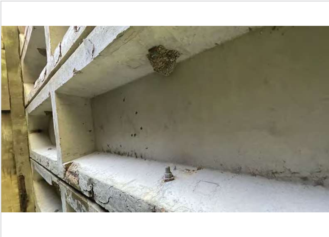
Bottom deck span #2 PCCS "F"
